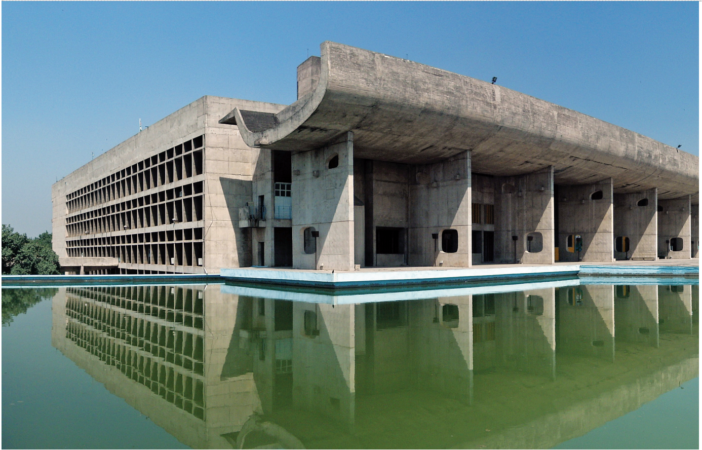
The Assembly building in the Capitol Complex of Chandigarh
